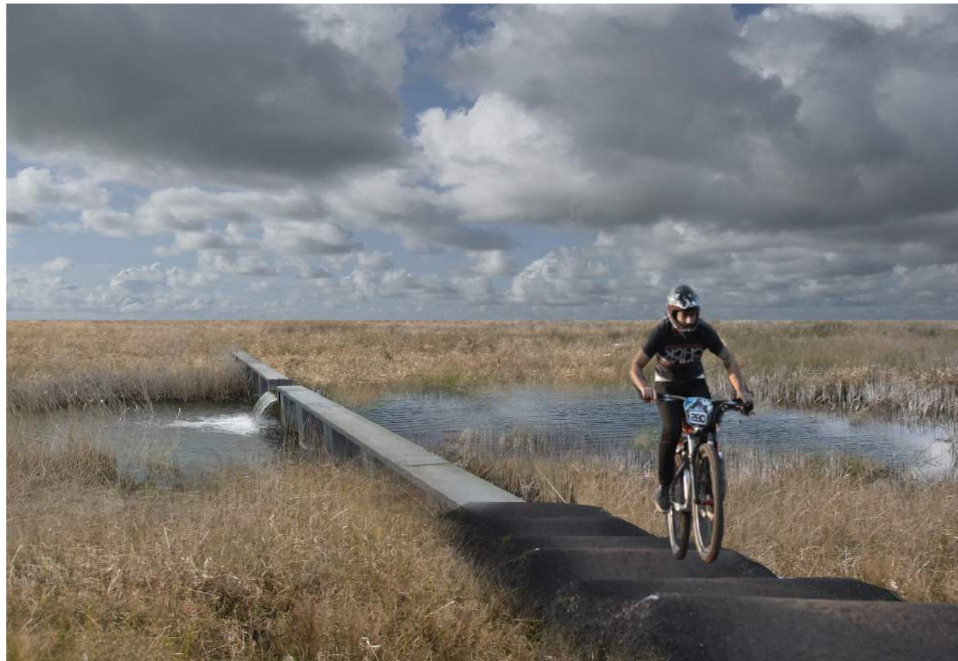
Figure 51. MERRITT CREEK PROJECT. Example of a combined water control and recreational amenity. This combined system improves water quality and reduces runoff, while providing an exciting experience for bikers.
