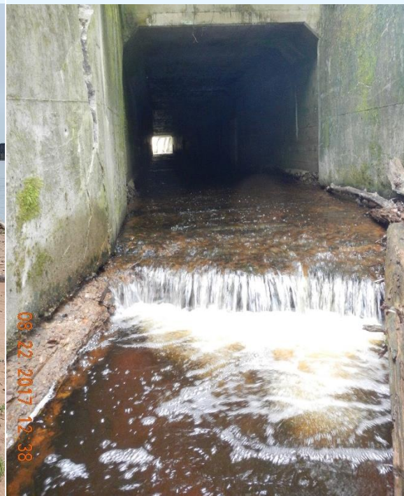
Final barrier at Little Balsam Creek
